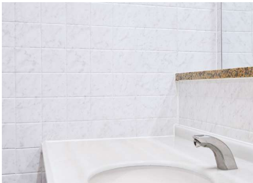
Restroom refurbishment / ST-024TIL
